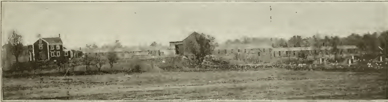
General View of Soft Roaster Plant of Henry D. Smith, Rockland, Mass.
